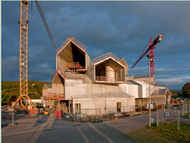
The VitraHaus by Herzog & de Meuron under construction
