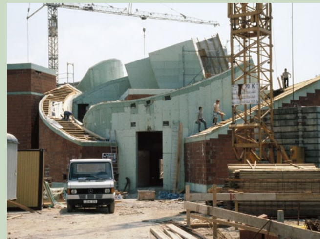
The Vitra Design Museum by Frank Gehry under construction
